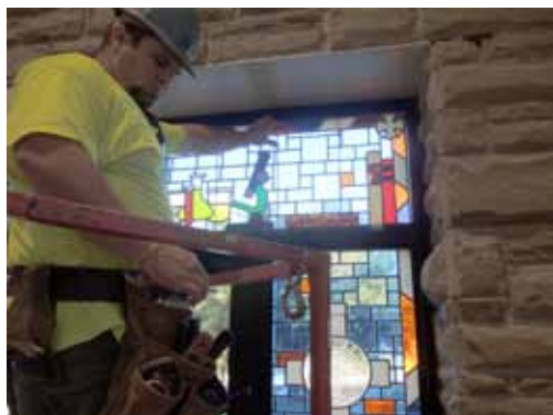
Installing stained glass in new entrance
