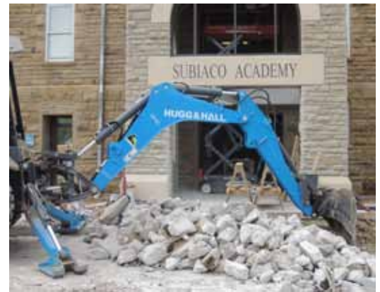
Front entrance under construction
