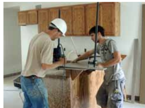
Carl Stengel '95 and son installing cabinets in Fuhrmann Hall
