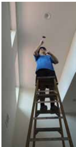
Installing access points in Fuhrmann Hall
