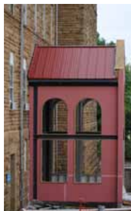
Progress on new front entrance
