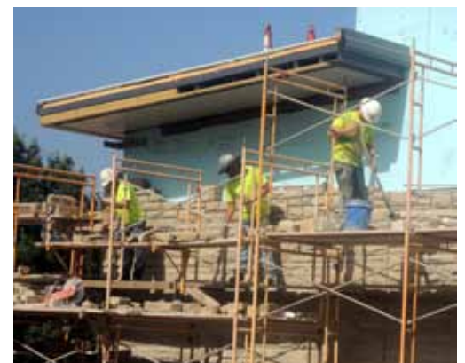
Stone masons at Fuhrman Hall
