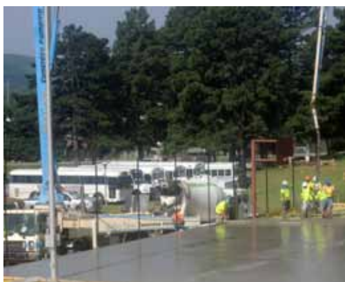
New tennis courts under construction
