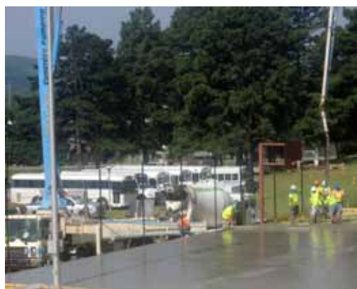
New tennis courts under construction
