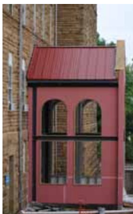
Progress on new front entrance
