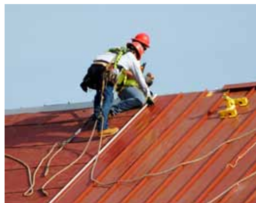
Roof on the Abbey church is nearing completion.
